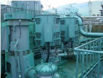
Unit1 PCV cooling sea water pump
