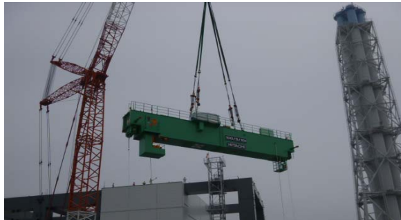
Overhead Cranes Brought in (On June 7)
