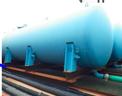
Steel horizontal tanks
