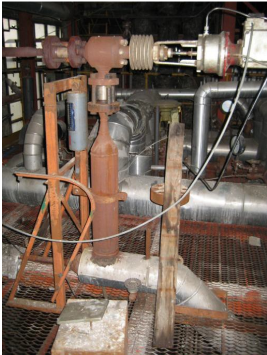
Pneumatic actuator of loop pressure control valve (V4 in Fig.2b).
